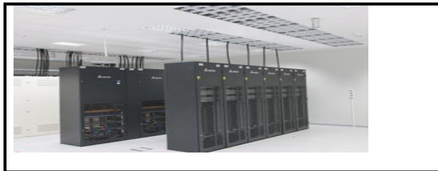
Gambar 3.25 Mobile Switching Center
