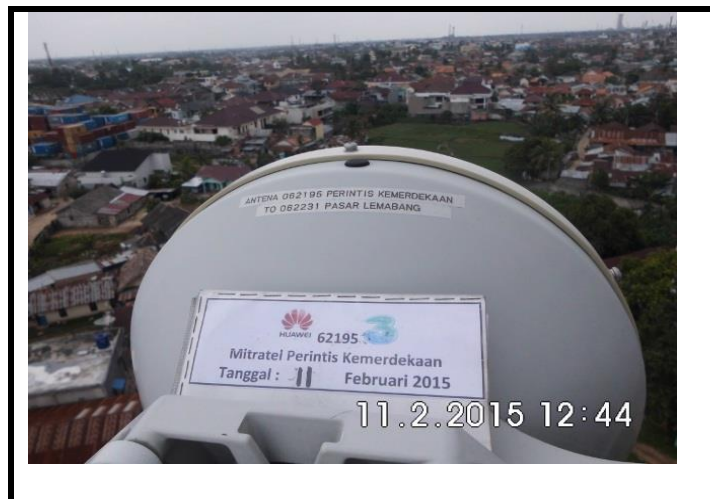
Gambar 3.5 Antena Microwave
