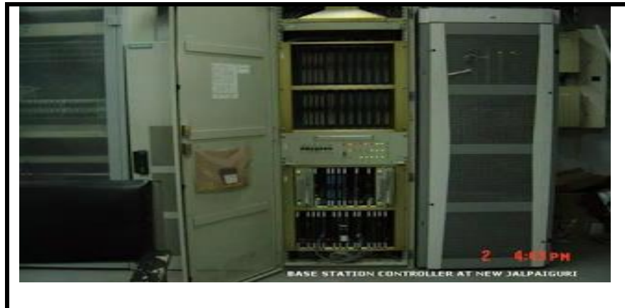
Gambar 3.26 Base Station Controller
