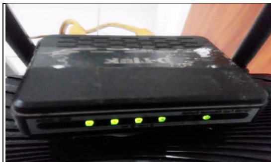
Gambar 3.3 Switch D-Link 8 port
