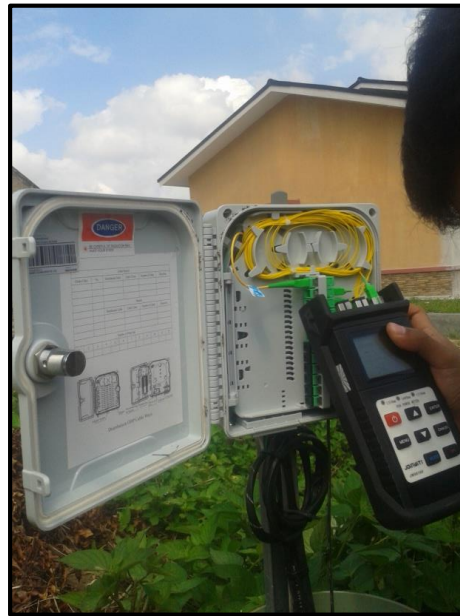
Gambar 3.6 Fiber Access Terminal Huawei GXF147-FAT2120TD-12
