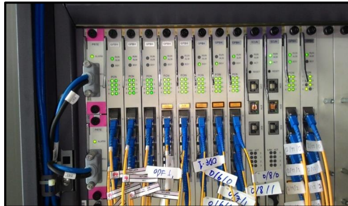
Gambar 3.3 Optical Line Terminal Huawei SmartAX MA5600T
