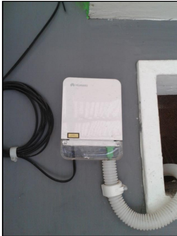
Gambar 3.7 Terminal Box Huawei ATB3101-1B
