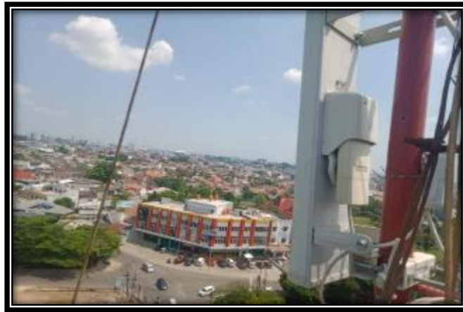
Gambar 3.9. Radio Rocket M5 Antena Sectoral AM-5G19-120 ( AccessPoint )
